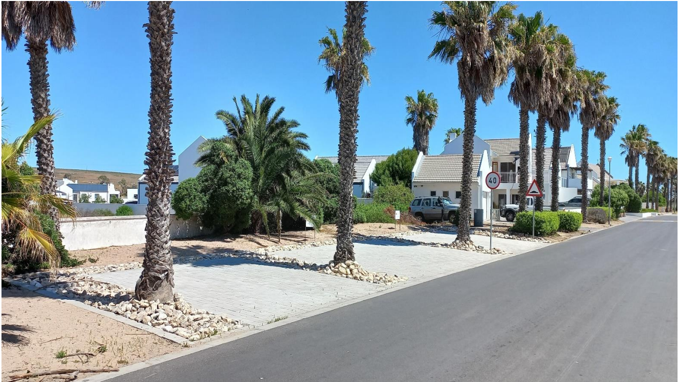
Completed Parking Bays and landscaping
